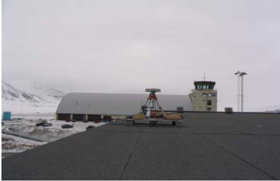
Figure 5.2-1 Longyearbyen: DGPS ground station, antenna on the roof of the hangar building. Receiver was installed in a separate room of the hangar. Data was named with LYR.
