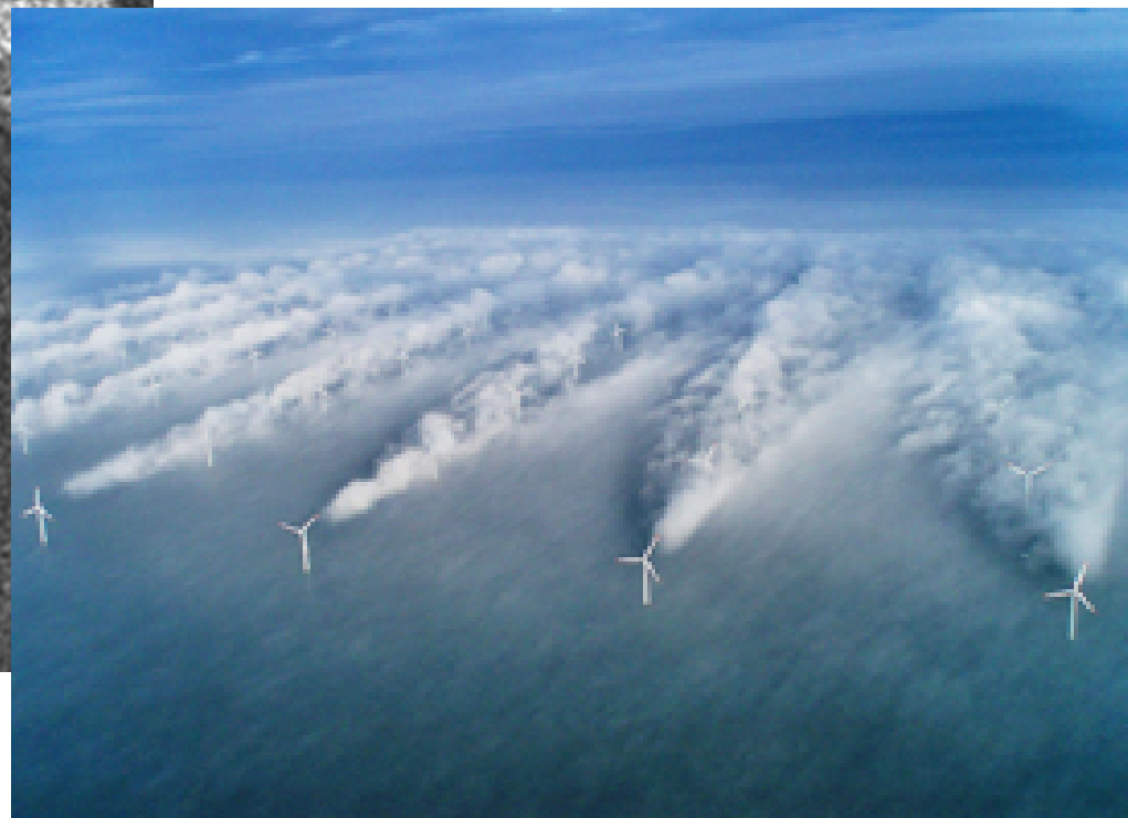
Wind wakes shown by clouds downwind of the Horns Rev offshore wind farm, Denmark
